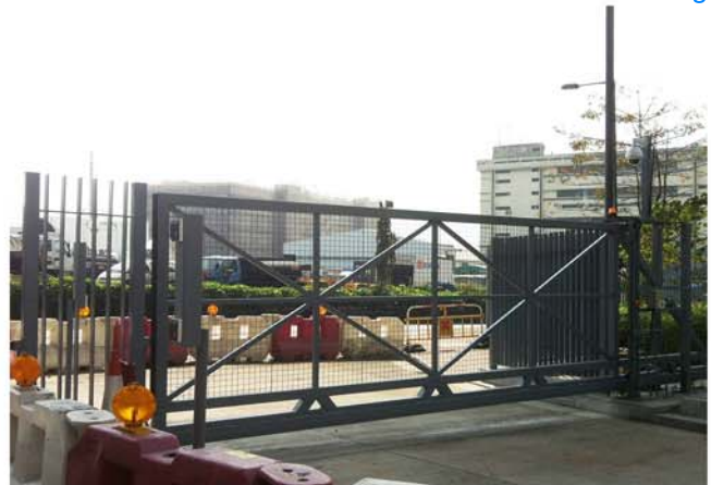
Completed with fencing & surveillance cam
